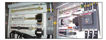
Wiring is permanently tagged and color coded for ready identification.
