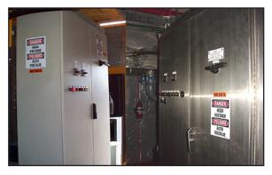
**Motor starter** and **controls** are contained in fiberglass or 316 stainless steel enclosures. The motor starter is a soft start type to reduce inrush current.
